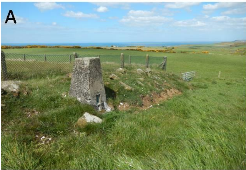
A. Scudion Craig trig pillar. B. Flush bracket on Scudion Craig trig pillar.
