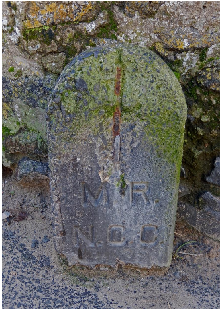
Detail of the MRNCC railway boundary stone. Some TLC is required.
