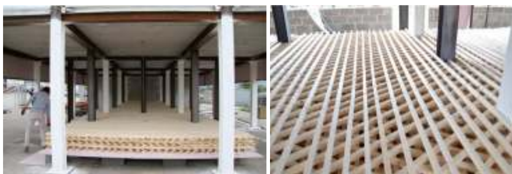
Figure 4. Fuel load arrangement and steel columns (with and without fire protection)
