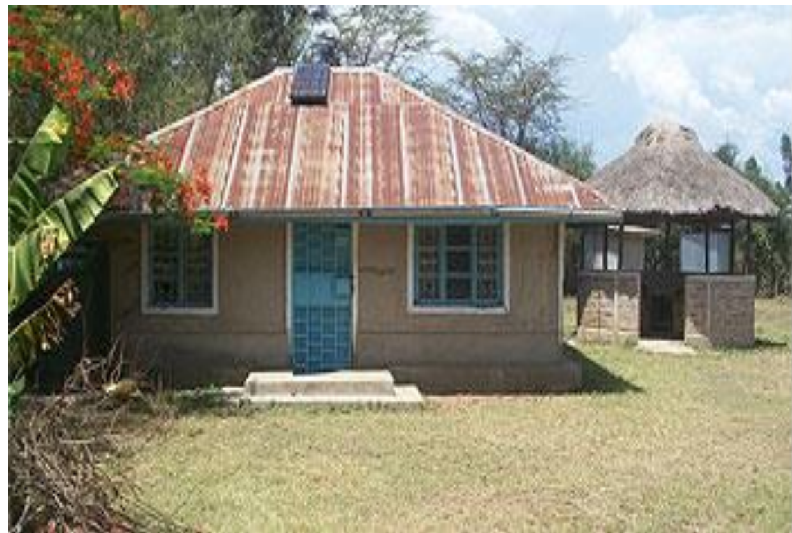
Fig. 1: A House with PV in Kendu Bay Area of Kenya
