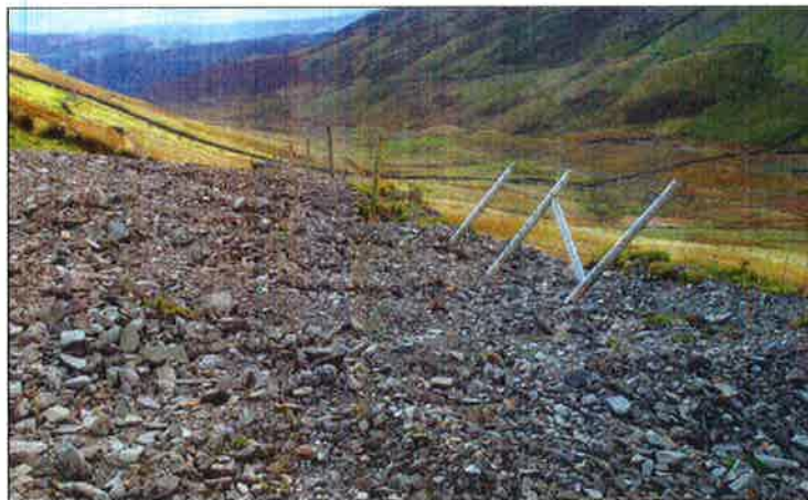
Figure 8. The debris of Fan 11 is level with the top of the wall and has spilt over into the enclosure. It has also disturbed the fence that was built to maintain the boundary and prevent sheep from jumping into the enclosure.
