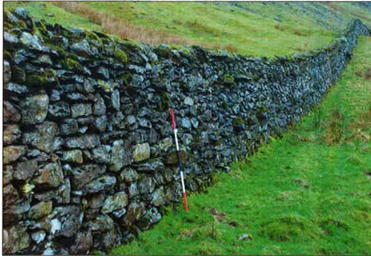
Figure 9. A section of the downslope-facing Dalehead Close wall with rows of projecting through stones at 0.5 m and 1.2 m above base. The survey pole divisions are at intervals of 0.2 m.
