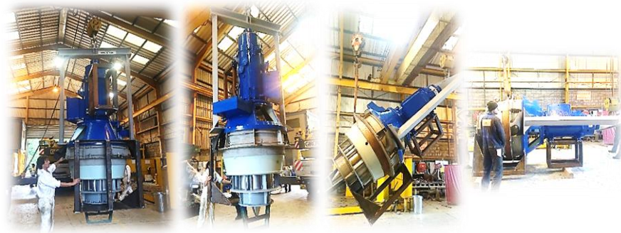
Figure 3: Lifting rig in operation
